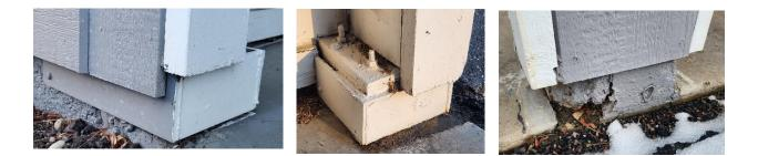
• New carport opening trim boards (2 x 8's) are re-installed to be flush with the siding and trim, and the trim is flashed to prevent future moisture intrusion. Metal L-brackets (often salvaged from the old trim boards) are attached to the 2 x 8's at car bumper height for reinforcement.
