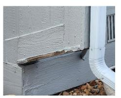
• Buckled or rotten siding due to sun or moisture is replaced. The wall of the B unit next to the A unit is frequently rotten. Unfortunately, the original building used 9 foot sheets of siding, and only 8 foot sheets are now available. So some horizontal joints (see photo below) are now required with proper flashing. OSB and/or Tyvek building wrap is installed under new siding.
