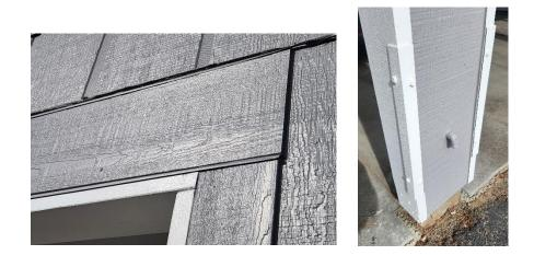
• The trash room door is often re-built, and the trim is re-done and properly flashed. The trash room door swing should be examined and changed if necessary so that it swings closed with the West or NW wind. New substantive hardware is required, secured with through-bolts, not just screws.
