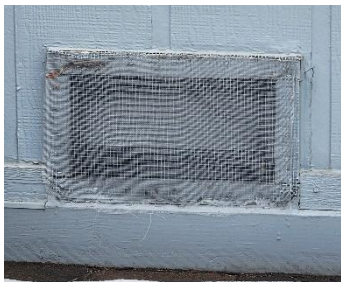
Inadequate crawl space vents In disrepair
