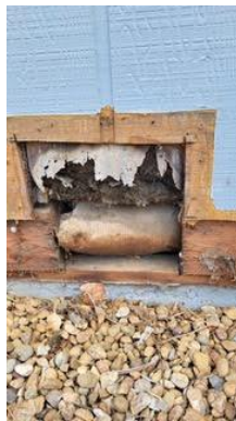
Inadequate crawl space vents In disrepair
