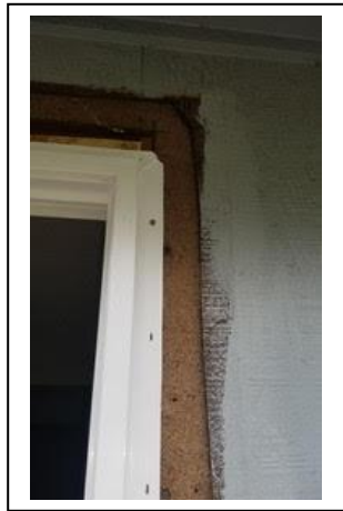
Window flanges & siding cut back
