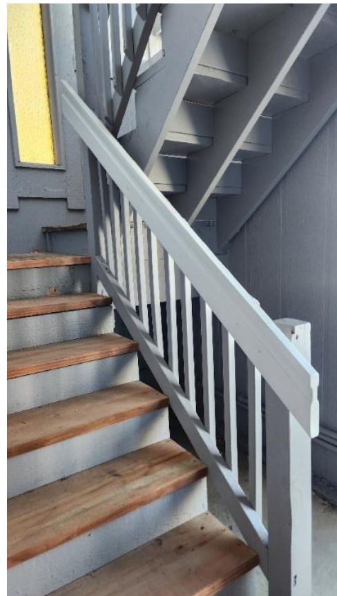
New stairs with three stringers and closed risers and proper balusters & handrail.
