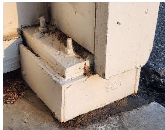
Repaired concrete piers
