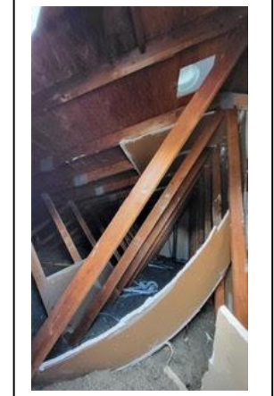
Fallen drywall in attics, crushing insulation
