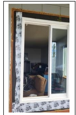
Flanges caulked & taped
