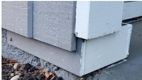
Repaired concrete piers
